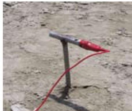
Earth Test Spike
