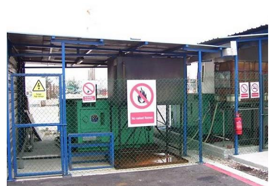
Fencing for a diesel generator installation
