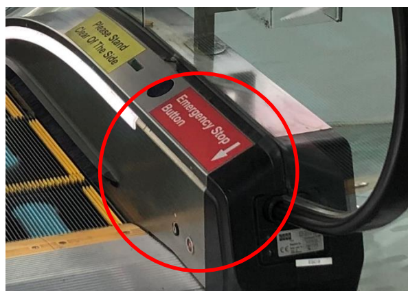
Emergency stop button with signage on escalator landing and mid-point (for longer escalators)
