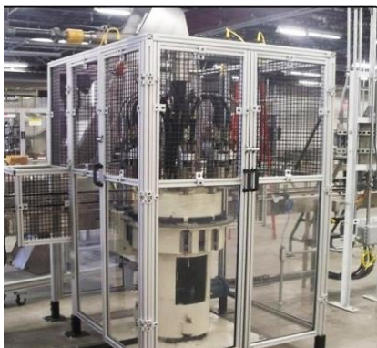
Suitable types of metal fencing and panel systems around energised equipment
