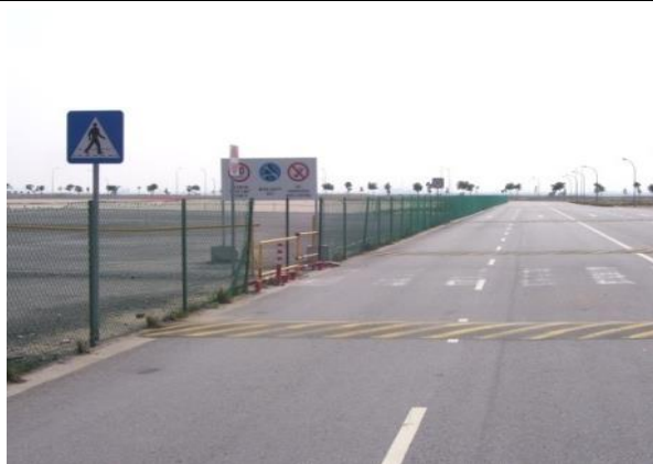
Speed bump and clear signage used to slow down vehicles approaching hazard areas
