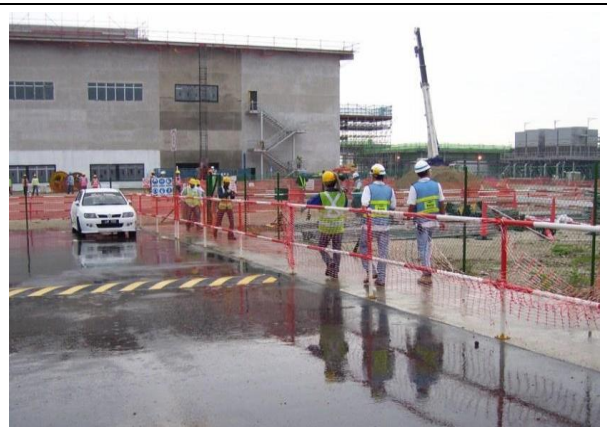
Barriers and guardrails erected to form separated pedestrian routes
