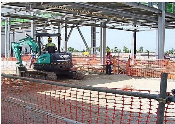
Robust exclusion zone established around earth moving machine; a banksman provides traffic marshalling during excavation operation
