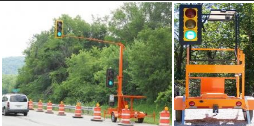
Use of traffic /portable lights versus traffic controllers at construction exit points
