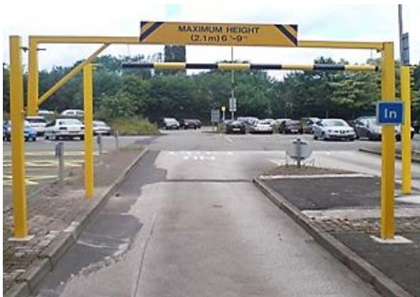
Example of height limit barriers
