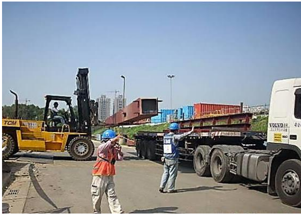
Trained traffic marshal/signallers guiding vehicular movement and loading/unloading activity.
