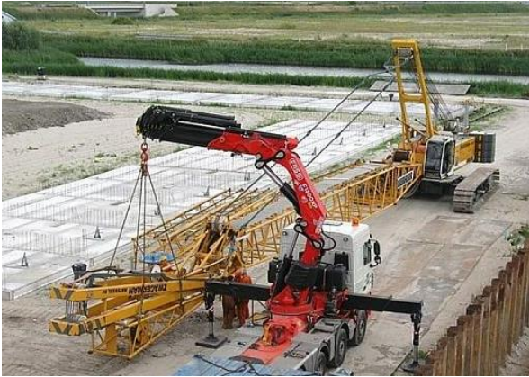
Installation/ Dismantling of plant and machineries at a safe location
