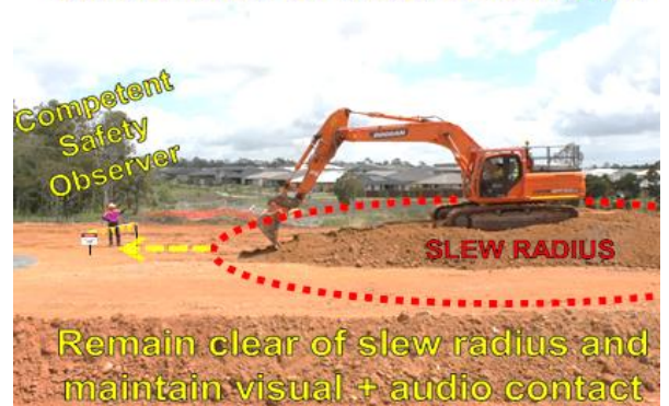
Excavation operation that observes clear space between man and machinery
