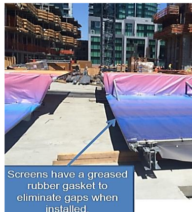
Screen panels arrive pre-assembled with rubber gaskets installed, ready to lift in place
