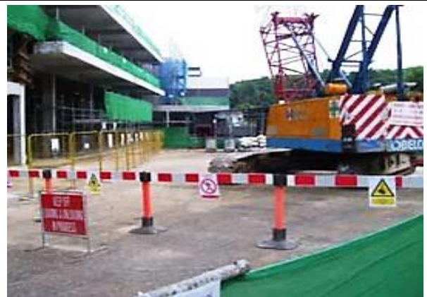
Exclusion zone established around lifting machine
