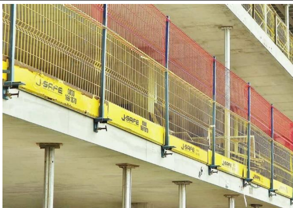
Examples of enclosures provided for work areas to prevent fall of persons and materials
