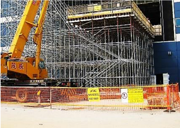
Exclusion zone established with hard barricades, safety mesh and signage, and large enough to accommodate the height from which material may fall.
