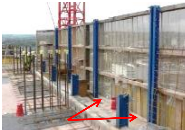
Gaps between climbing screen and construction floor sealed to comply with Lendlease's "No Gap" policy
