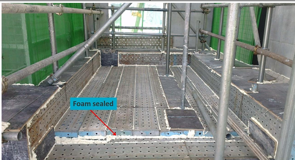
Gaps on work platform foam sealed to prevent materials from falling through
