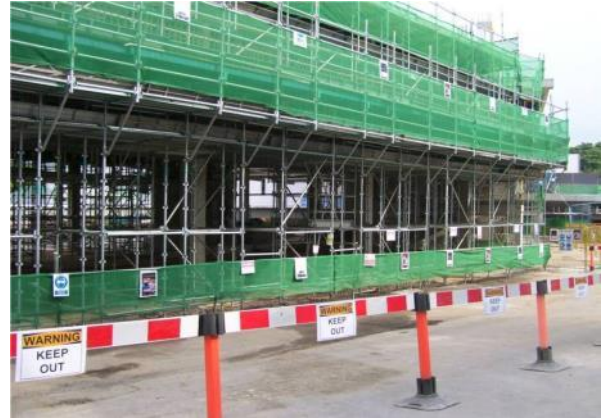
Collective exclusion zones in the form of robust guardrails with netting plus bollards and planks extending far enough and with visible signage.
