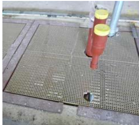
Mesh cut just enough to fit riser
