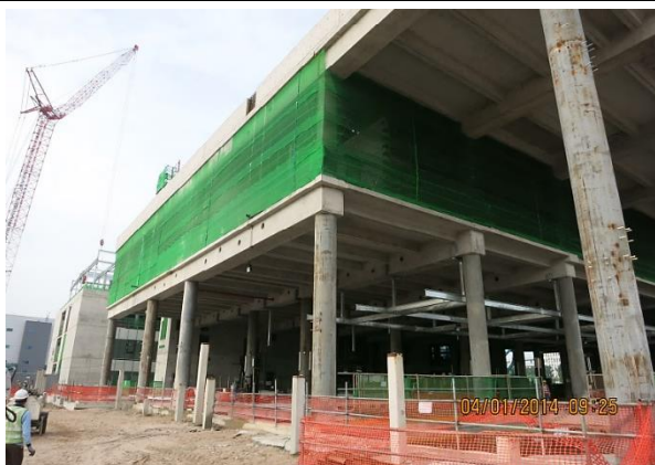
Fully enclosed edge protection consisting of robust guardrails and full height netting
