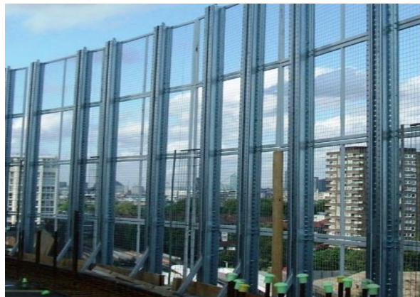
View from internal of perimeter screen
