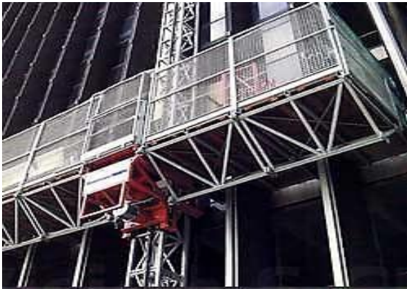
Mast climbing work platforms installed with mesh or nets to provide protection for fall of persons and materials
