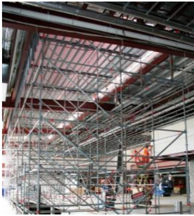
Birdcage scaffold using proprietary scaffold system
