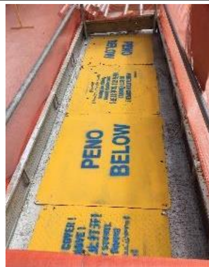
Examples of floor penetration covers firmly secured
