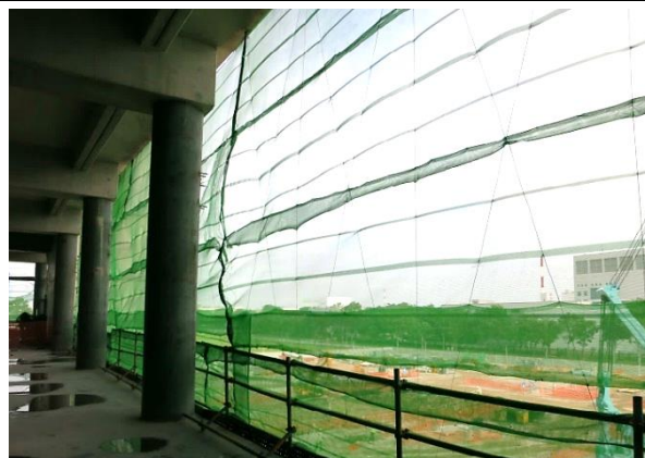
Fully enclosed edge protection consisting of robust guardrails and full height netting
