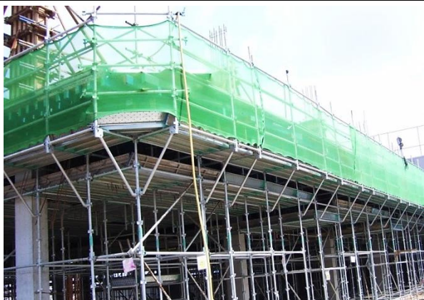
Provision of perimeter edge protection and good work access at slab edge as part of falsework system
