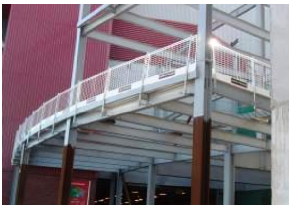
Proprietary edge protection system provided during steel structure installation
