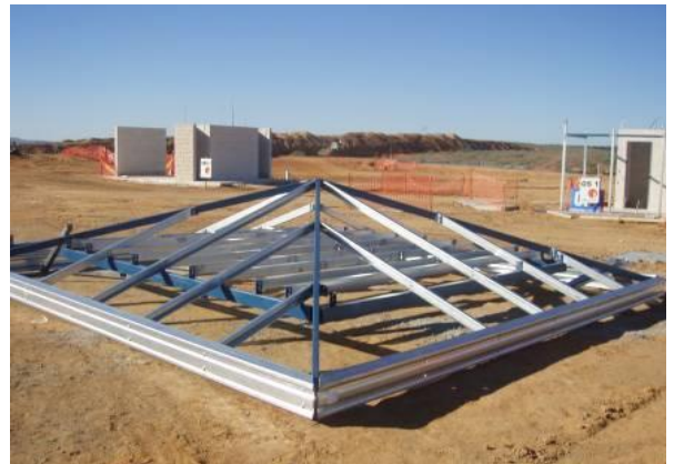
Pre-fabrication of roof structure on ground
