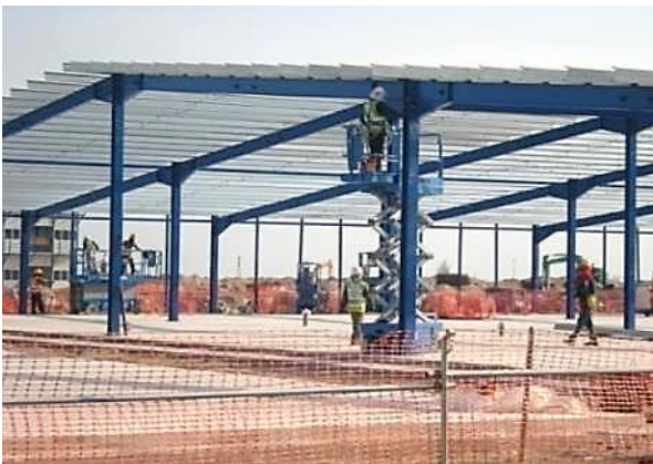
Steel erection using scissor lift within an exclusion zone
