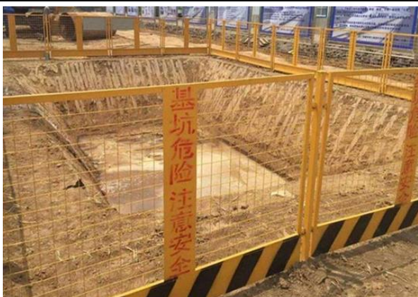
Excavation edge protection barriers
