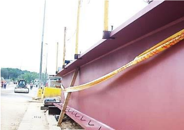
Stanchions with lifeline fitted to beam before lifting
