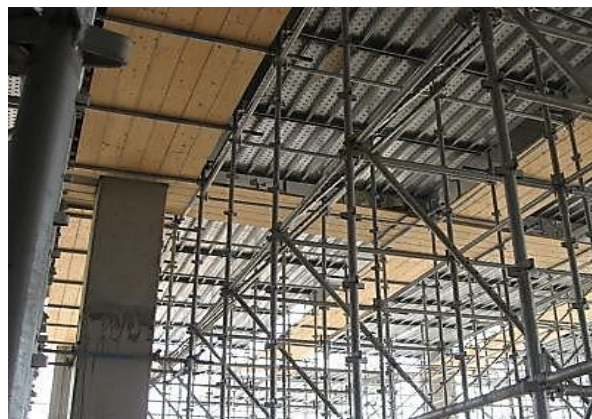
False work with a full deck to allow installation/dismantling of formwork from below
