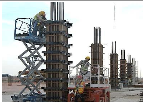
MEWP access for column work
