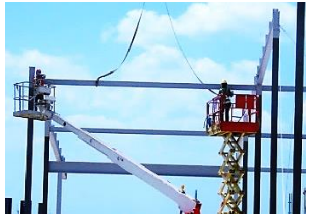
Collective use of boom lift and scissor lift
