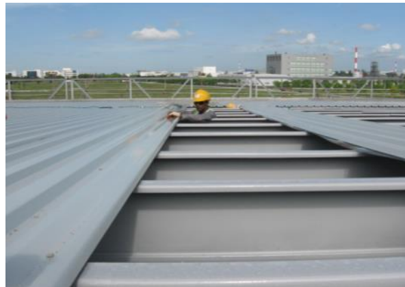
Roof sheets installed from a MEWP
