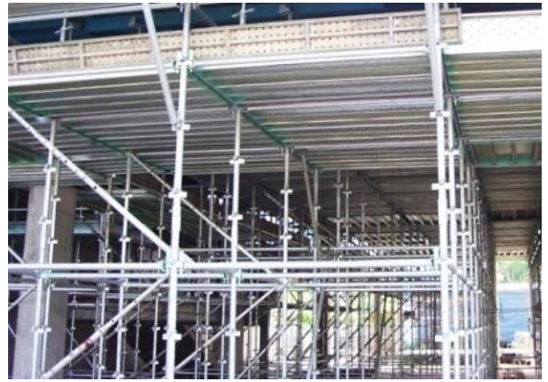
Birdcage scaffold with a working deck for installation/dismantling of formwork from below
