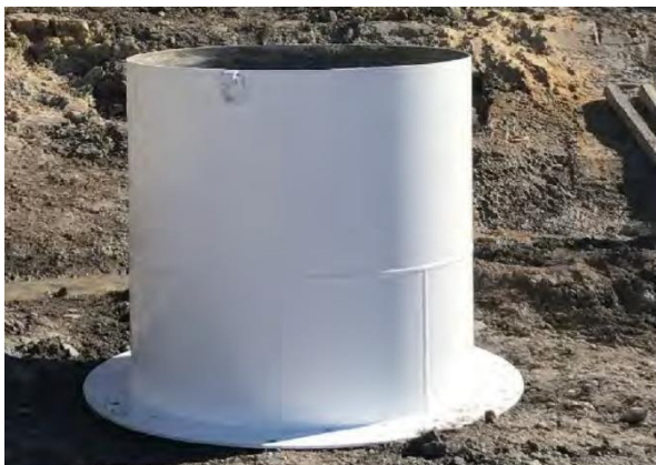
Extended pile casing to offer fall protection
