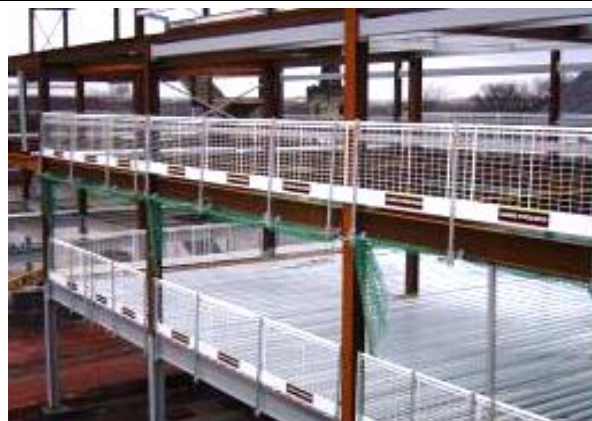
Proprietary edge protection system provided during steel structure installation
