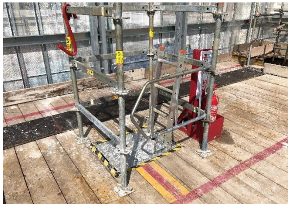
Examples of safe access (internal) provided to working deck of core
