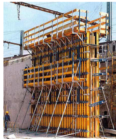
System formwork used for RC wall construction
