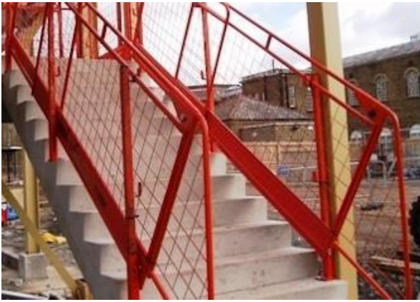
Permanent stairs with temporary barriers to provide fall protection
