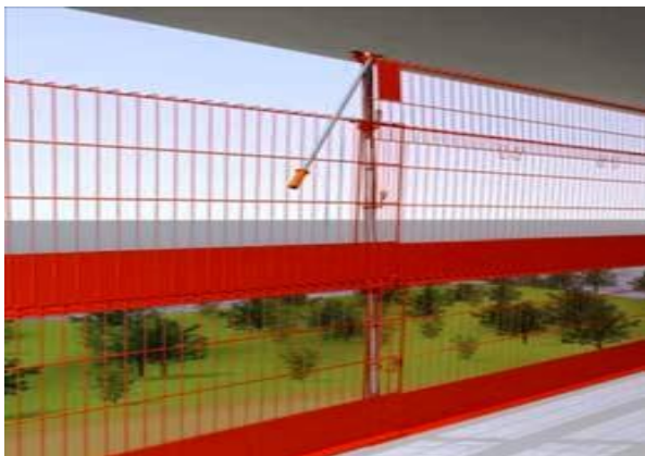
Adjustable full height proprietary edge protection system to provide access for subsequent works, e.g. façade fixings.
