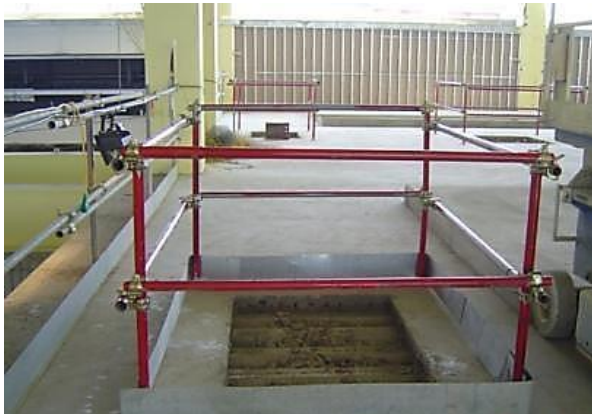
Hard rails and toe boards installed before cutting out mesh
