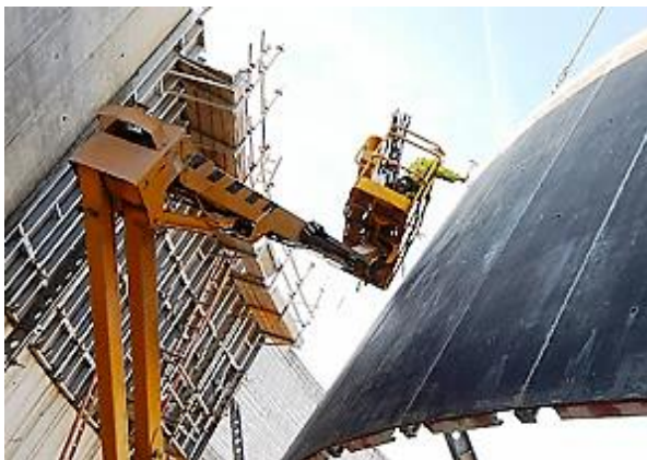
Prefabricated wall formwork lifted into place and installed with telescopic boom lift
