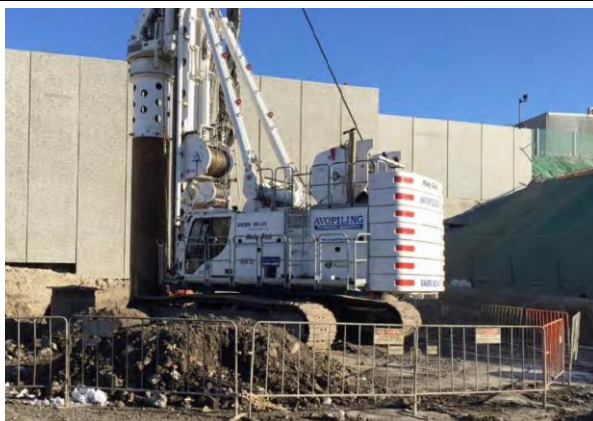
Fences installed to act as exclusion zone barriers during boring works
