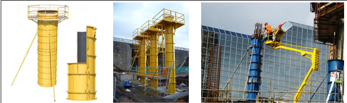
Circular/round column formwork with safe access platforms or access via articulated boom lift
