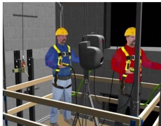
Work platform or elevator false car with guardrails provides safe work environment for installers within elevator shaft
