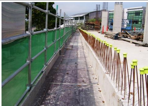
Provision of perimeter edge protection and good work access at slab edge as part of falsework system
