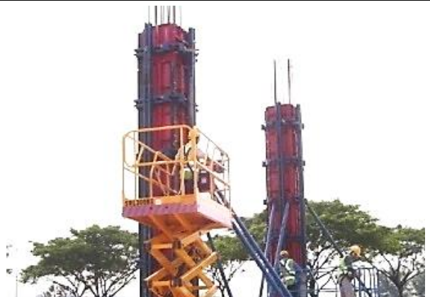
Column formwork closure with scissor lift
