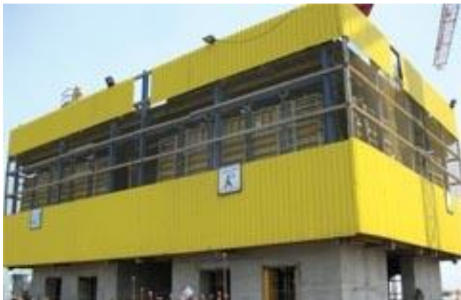
Self-climbing (ACS) core formwork system
