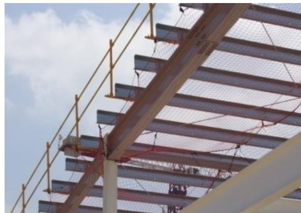
Perimeter edge protection and safety net
