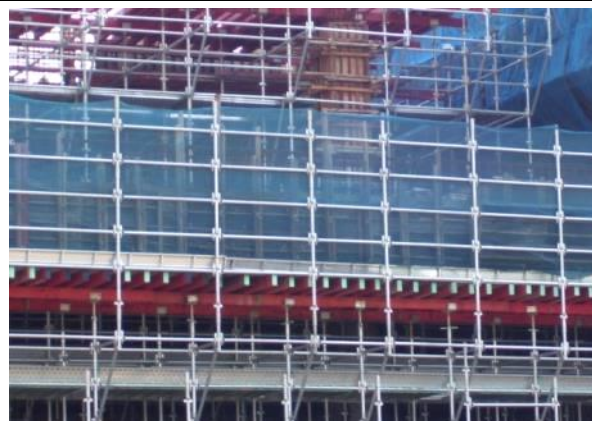
Perimeter edge protection on construction deck using proprietary scaffold system with multiple rails, toe boards, floor to top rail netting (>1.8m)
