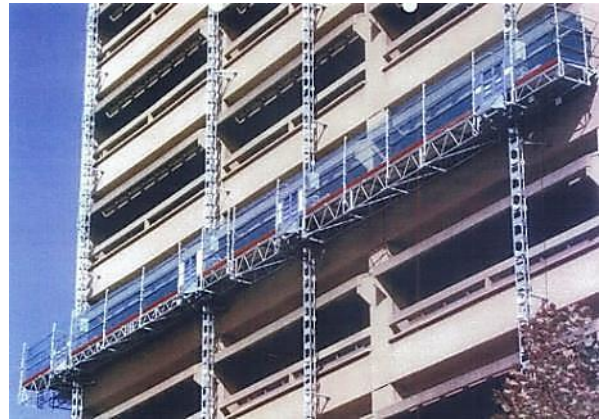
Mast climbing work platforms installed with mesh or nets to provide protection for fall of persons and materials
