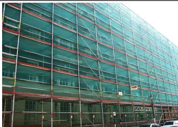
Proprietary perimeter scaffold with netting
