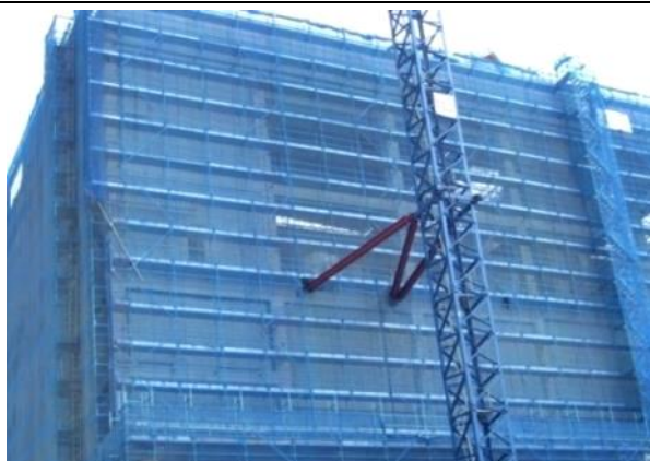
Perimeter scaffold with netting
