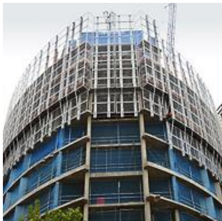
Examples of perimeter screens providing effective edge protection
