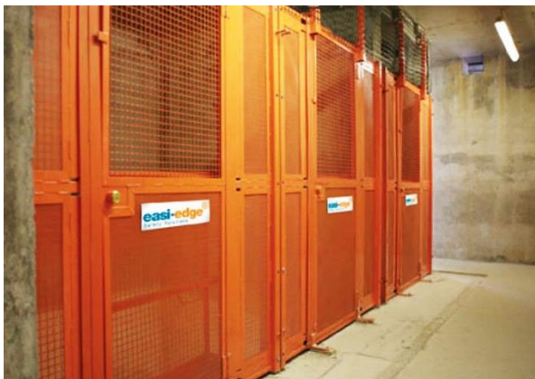
Full-height lockable gate system for lift shaft management
