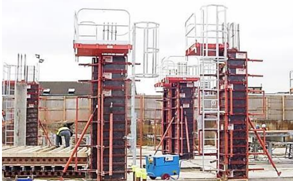
Proprietary column formwork providing safe caged access and working deck
