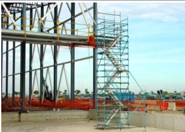
Stair access to steel deck
