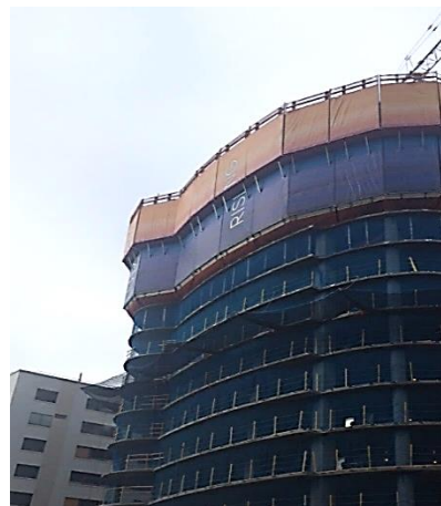
Examples of perimeter screens providing effective edge protection
