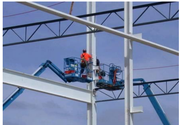
Bolt up from a Mechanical Access System
