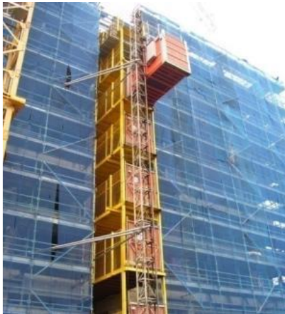
Single-cage passenger hoist
