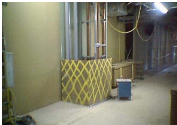
Services riser opening protected with 1.2m high 18mm protective board
