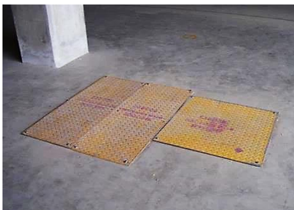
Examples of floor penetration covers firmly secured
