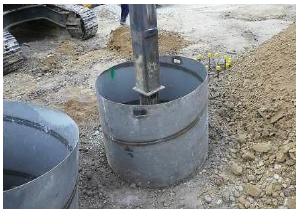
Caisson driven with its remaining portion (min. 1.2m high) left to provide edge protection to the bore hole
