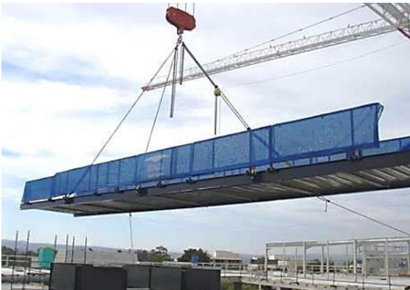
Pre-installed edge protection lifted in place
