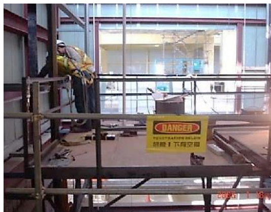
Work platform or elevator false car with guardrails provides safe work environment for installers within elevator shaft
