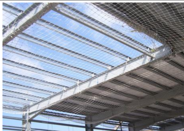
Perimeter protection and safety nets provided prior to roofing works commencing
