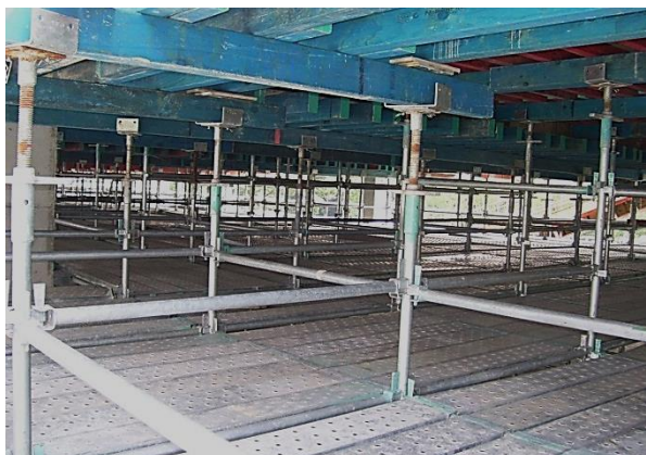
False work with a full deck to allow installation/dismantling of formwork from below
