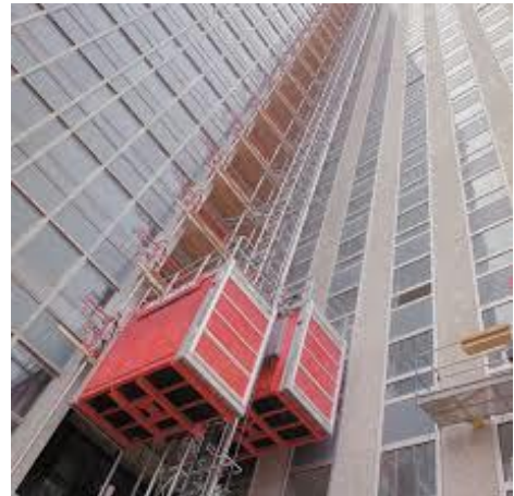
Twin-cage passenger hoist
