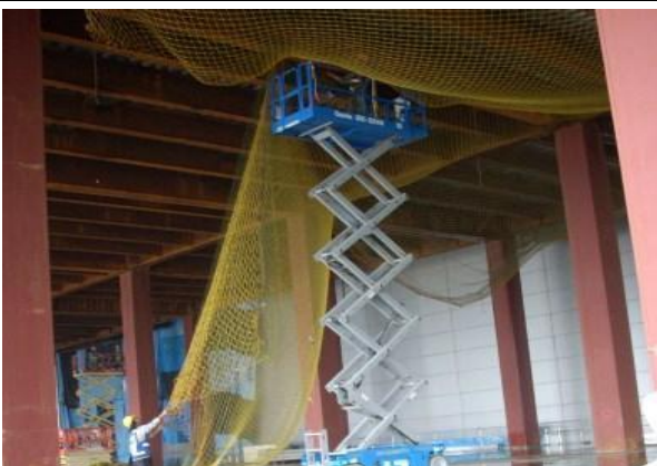
Safety nets installed and dismantled from MEWP
