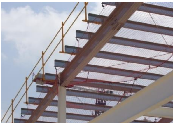
Perimeter protection and safety nets provided prior to roofing works commencing
