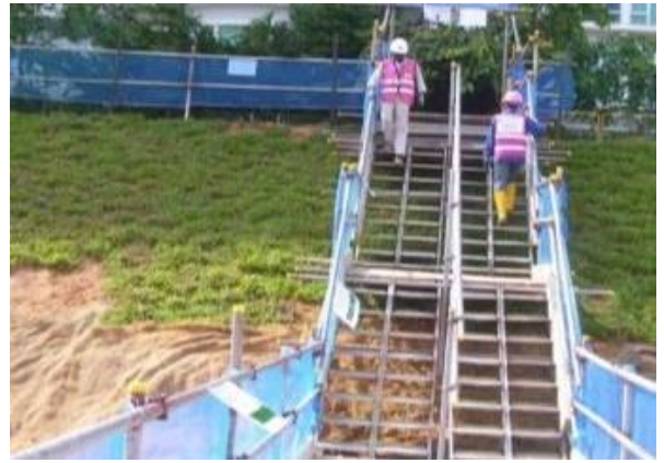
Temporary stairs of tube and fitting construction
