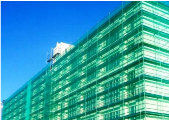
Face scaffold along perimeter of building fully planked, with handrails, bracings, toe boards and compliant stair access, and fully netted
