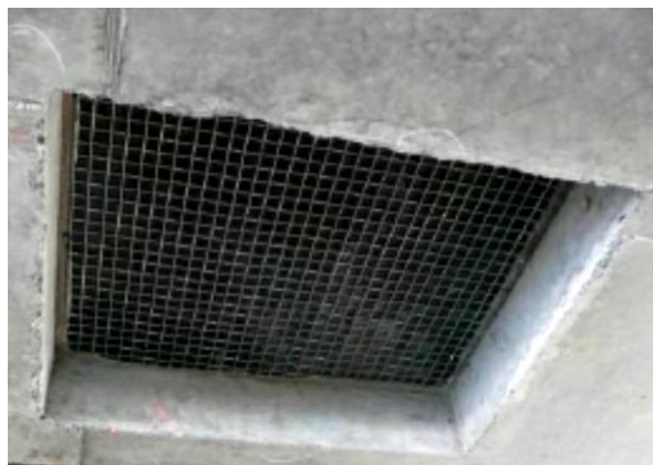
Medium penetration mesh cast in with secured cover on top
