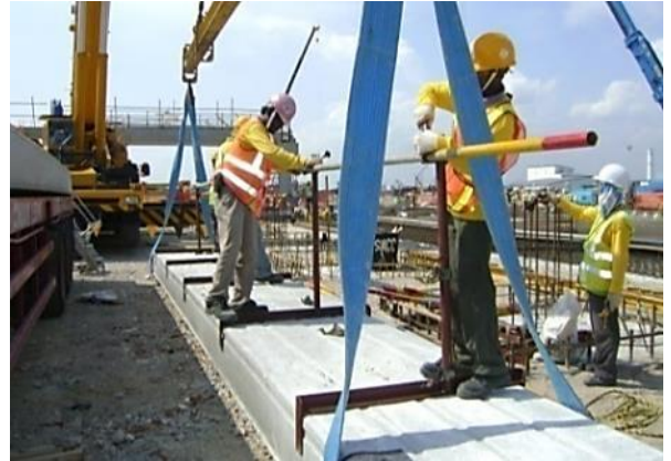
Pre-installed handrail edge protection on pre-cast RC slab section prior to lifting in place
