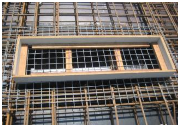
Mesh installed prior to slab casting
