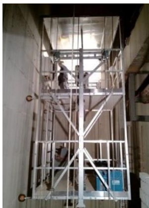
Work platform or elevator false car with guardrails provides safe work environment for installers within elevator shaft
