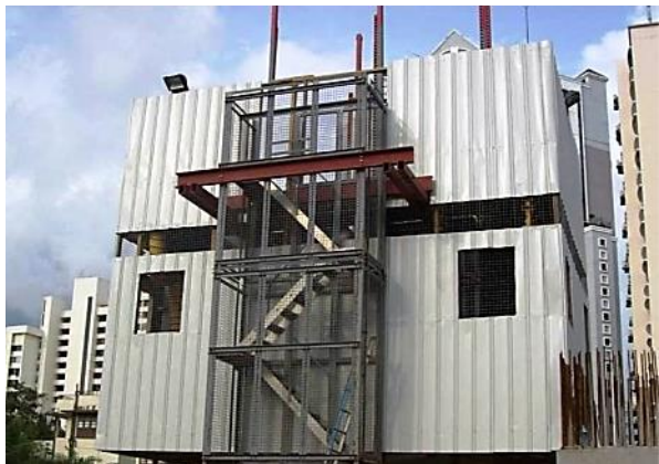
Safe access (external) provided to working deck of core
